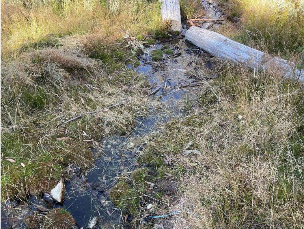
Photo 3 – concentrated water flow in boggy section of track
